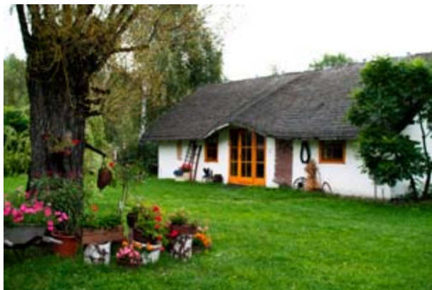
Photo 111. Traditional building in Sycówka. From the archive of LGD "PRYM".
