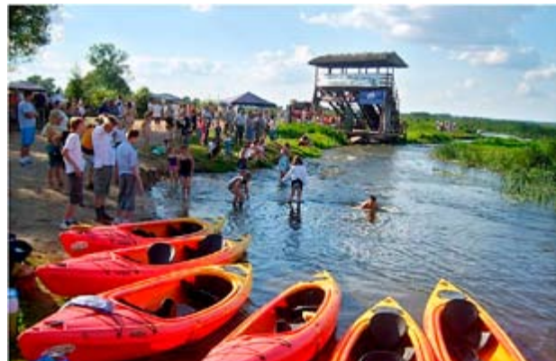
Photo 251. The lookout tower in Waniewo situated on River Narew. From the archive of LAG „N.A.R.E.W.”
