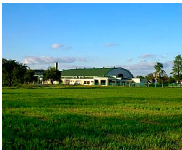
Photo 104. Sport and recreational infrastructure in LAG area. From the archive of LGD Tradycja, Kultura, Rozwój.
