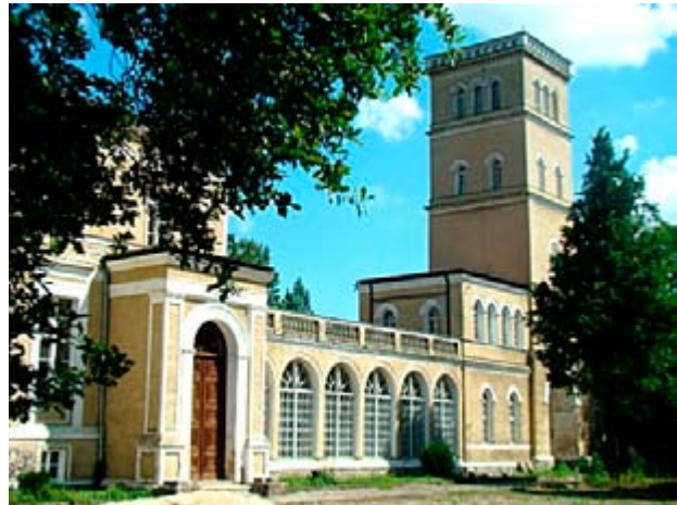
Photo 368. Palace in Strzelce. Source – From the archive of Municipal Office of Chodzież.
