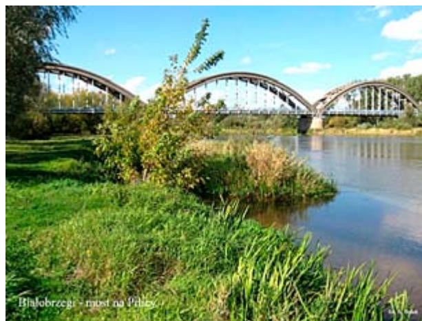
Photo 164. A bridge over the Pilica River in Białobrzegi, author: A. Bolek.
