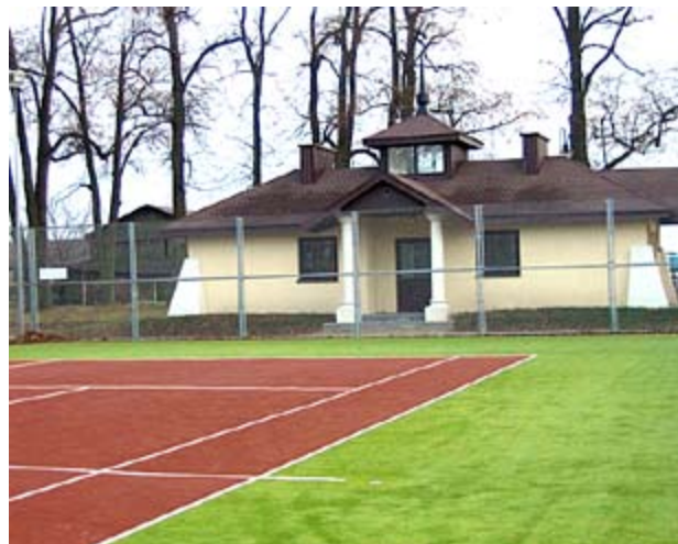
Photo 103. Sport and recreational infrastructure in LAG area. From the archive of LGD Tradycja, Kultura, Rozwój.
